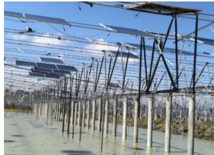
Figure 1. Field photograph of wind-induced damage to the cable-supported PV system. (Photographed by the author at Hainan, China).
